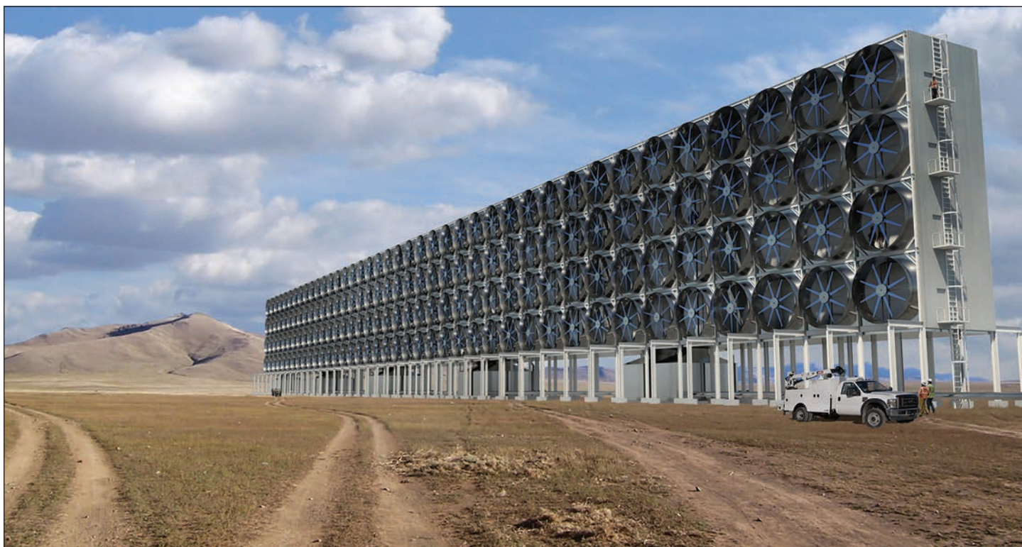
A rendering of Carbon Engineering's air scrubber. Each slab shown here can remove 100,000 tons of CO 2 from ambient air per year. Accompanying regeneration facilities then produce pure CO 2 for underground injection or use in making carbon-neutral transportation fuels. (Carbon Engineering photo)
