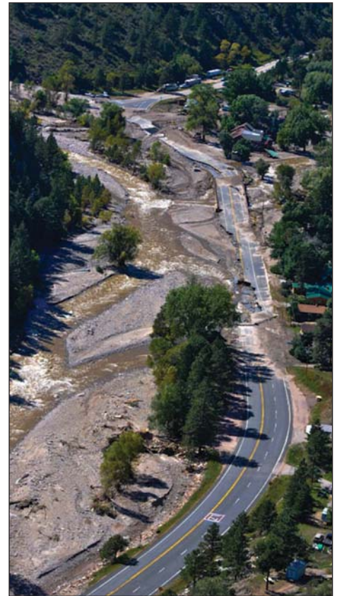
Devastation and destruction caused by the September 2013 flood in the Big Thompson Canyon near Drake, CO.
