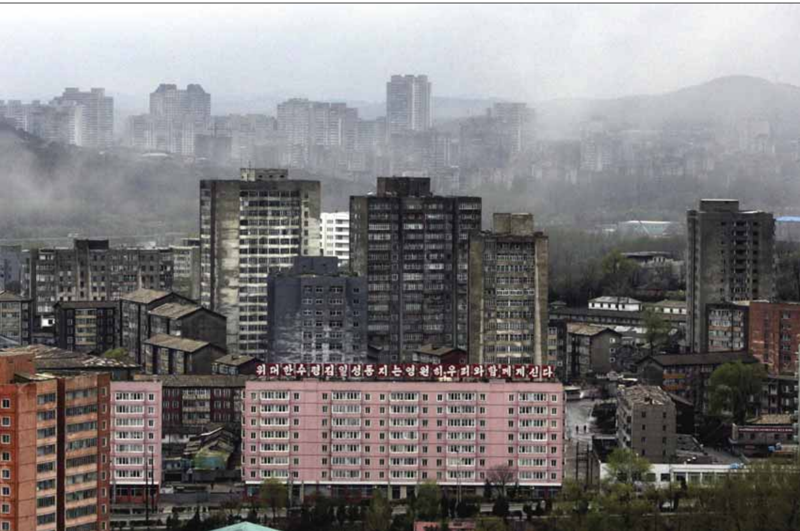
Need Reform. Smog-draped apartment buildings in Pyongyang, North Korea, greet South Korean delegates to an April 2007 meeting of an inter-Korean economic cooperation committee. Participants discussed aid possibilities despite North Korea's failure to make progress on an international agreement to dismantle its nuclear programs. (AP Photo/Park Min-kue, Korea Pool)
